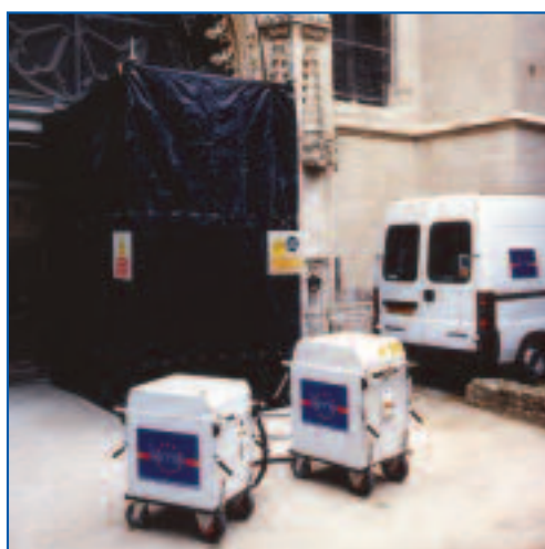
Figure 20 Use of opaque plastic sheeting to create controlled area for laser cleaning work outdoors.
