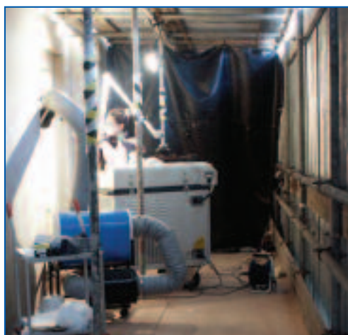
Figure 22 Laser cleaning within controlled area on scaffolding on St. George's Hall, Liverpool. Note use of opaque sheeting to divide laser work area from non-laser work area. All conservators on scaffolding wore laser safety eyewear whilst laser cleaning was carried out.
