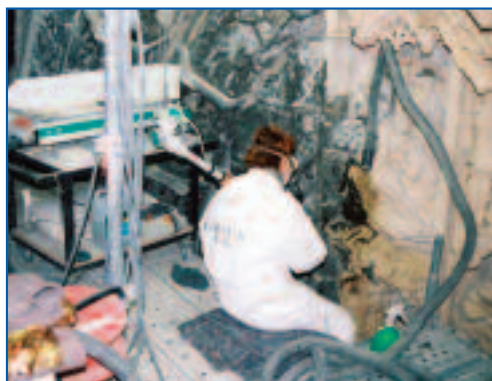
Figure 19 Laser cleaning within enclosed area on scaffolding on the exterior of Chapelle du Saint-Esprit, France.
