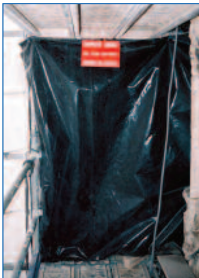
Figure 18 Use of opaque black plastic sheeting to separate laser work area from non-laser work area on scaffolding on the exterior of Chapelle du Saint-Esprit, Rue, France. Photo courtesy Quélin, France.
