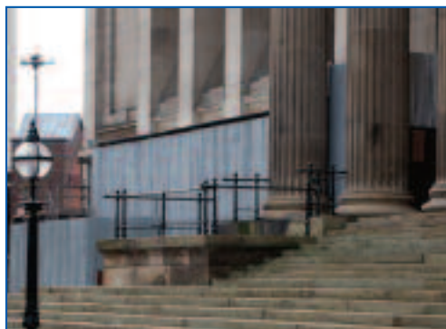
Figure 21 Use of tin hoarding on scaffolding to create safe area for laser cleaning on the outside of St. George's Hall, Liverpool.
